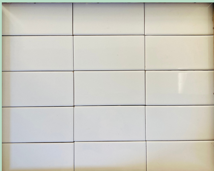
HORIZTONTAL STACK / STACK BOND
